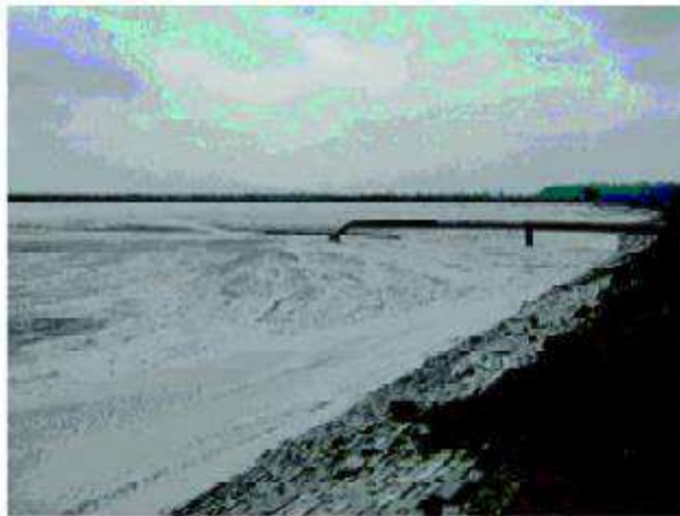
b) Safe Disposal for Control of Fugitive Dust with Uniform Discharge and Free Board
